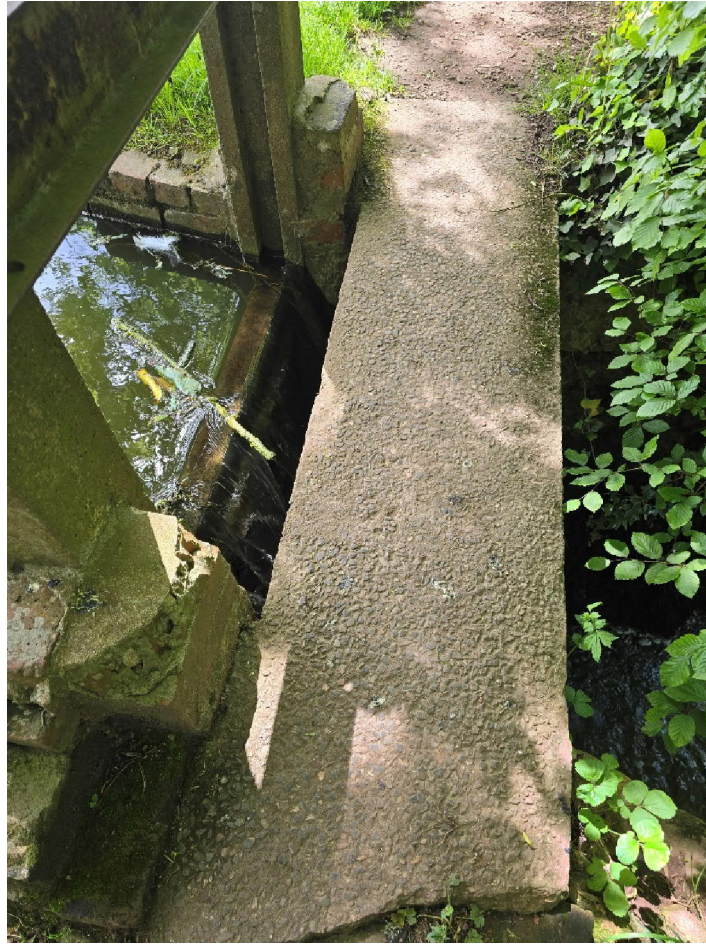
Sluice gate to south of bridge
