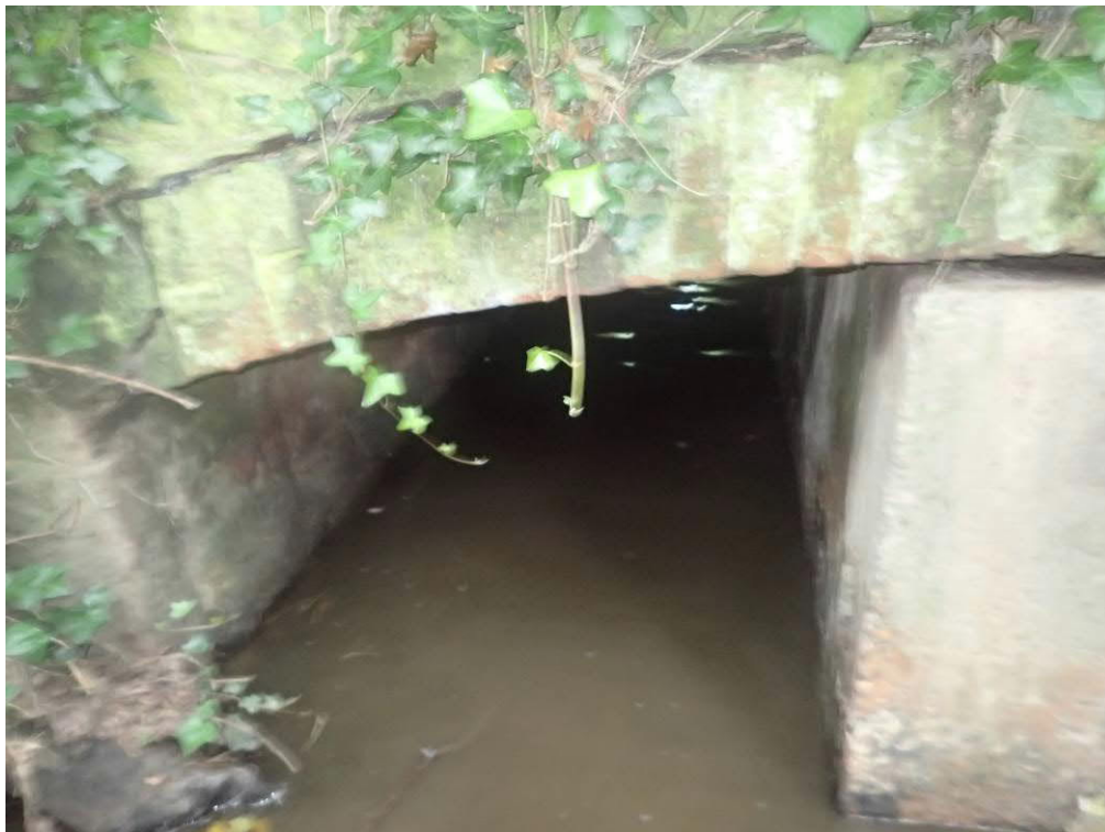
Photo 6 shows the inlet to the right culvert
