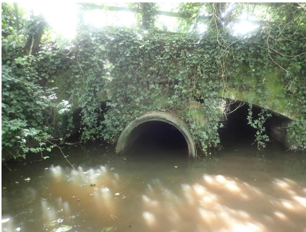
Photo 1 shows the downstream elevation of the bridge
