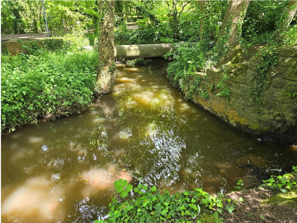
Pipe bridge and mill leats to south of bridge
