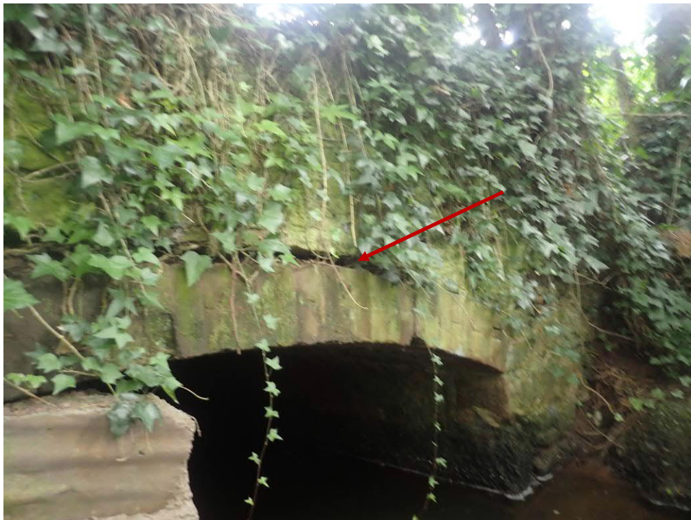
Photo 10 shows the dropped arch, viewed from upstream
