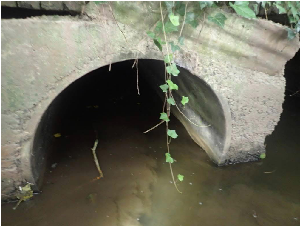
Photo 8 shows a view of the inlet to the middle culvert
