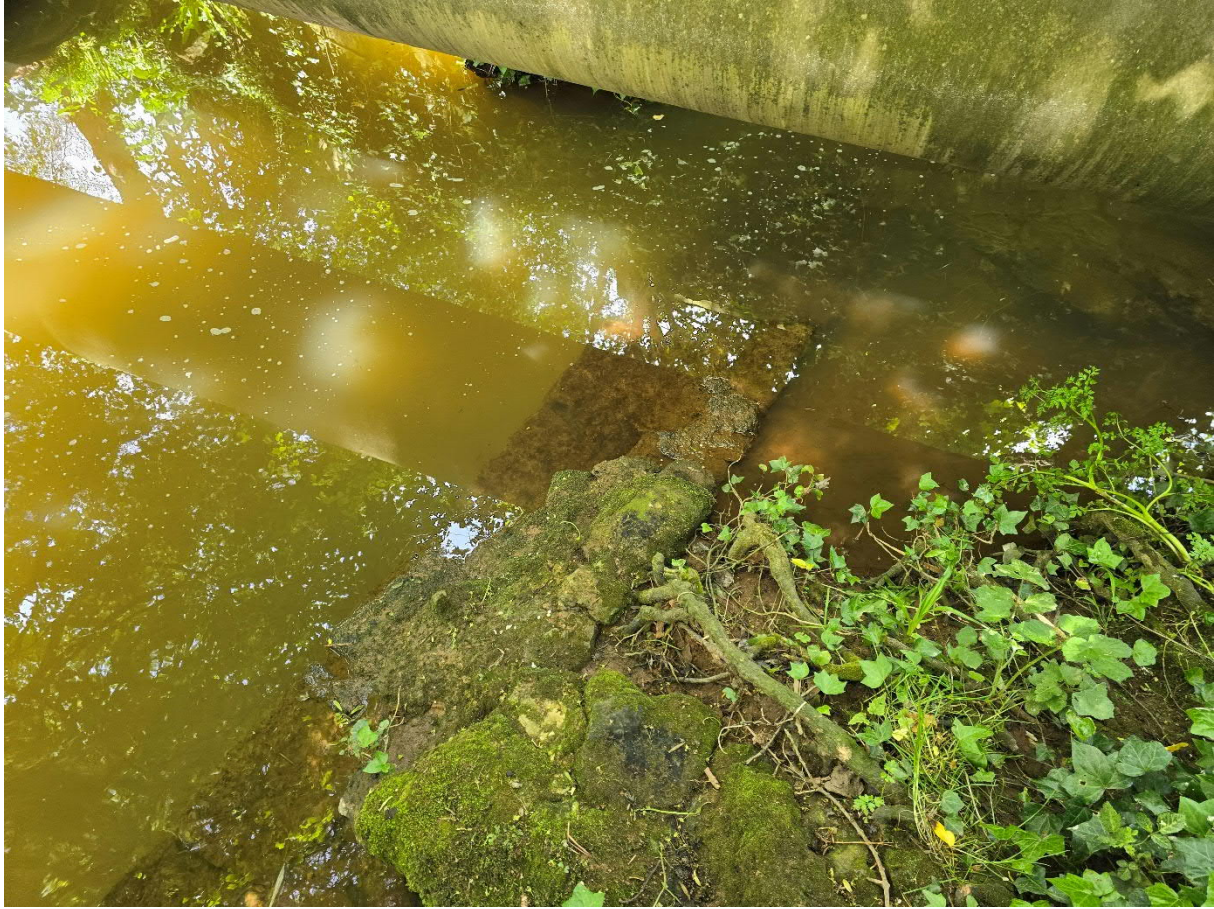
Partially submerged canalising wall to south of bridge
