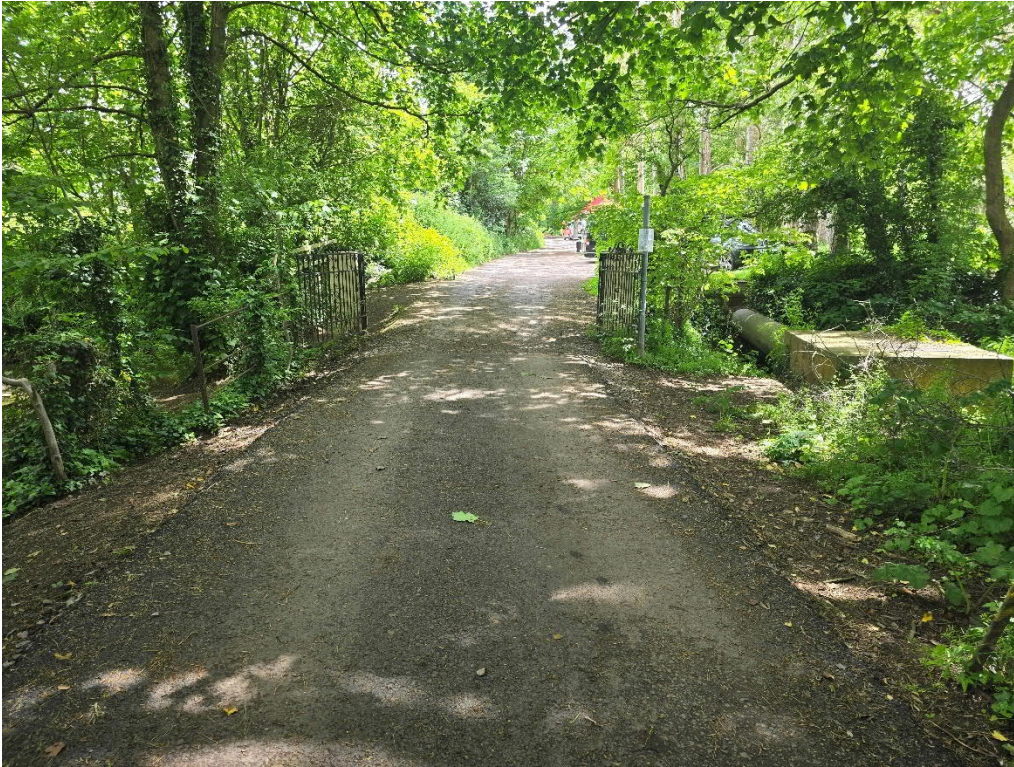
Figure 7: West looking east along bridge.
