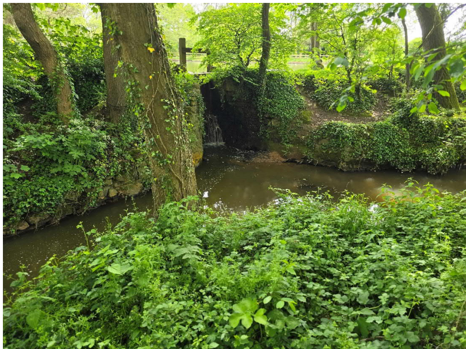
Sluice gate to south of bridge
