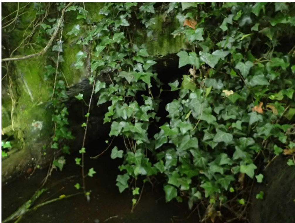
Photo 11 shows a view of the left culvert outlet
