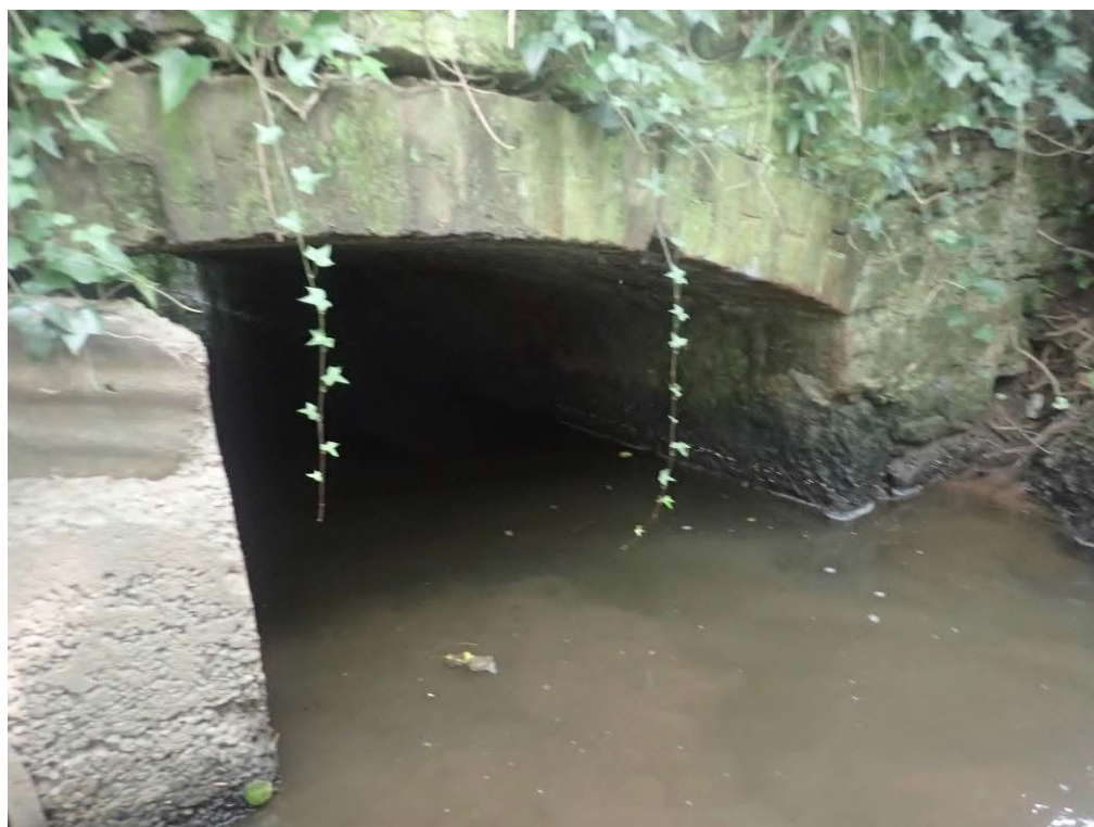
Photo 15 shows a view of the left culvert inlet
