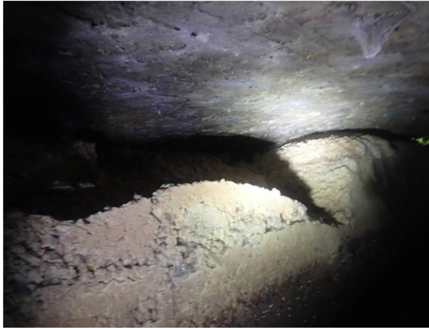
Figure 11: Photo extract from 2017 inspection report showing concrete to right abutment and bridge soffit.
