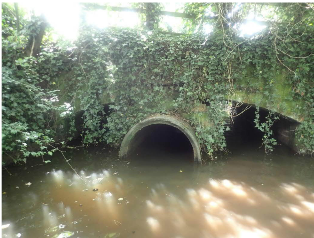
Figure 1: Downstream elevation of the bridge
