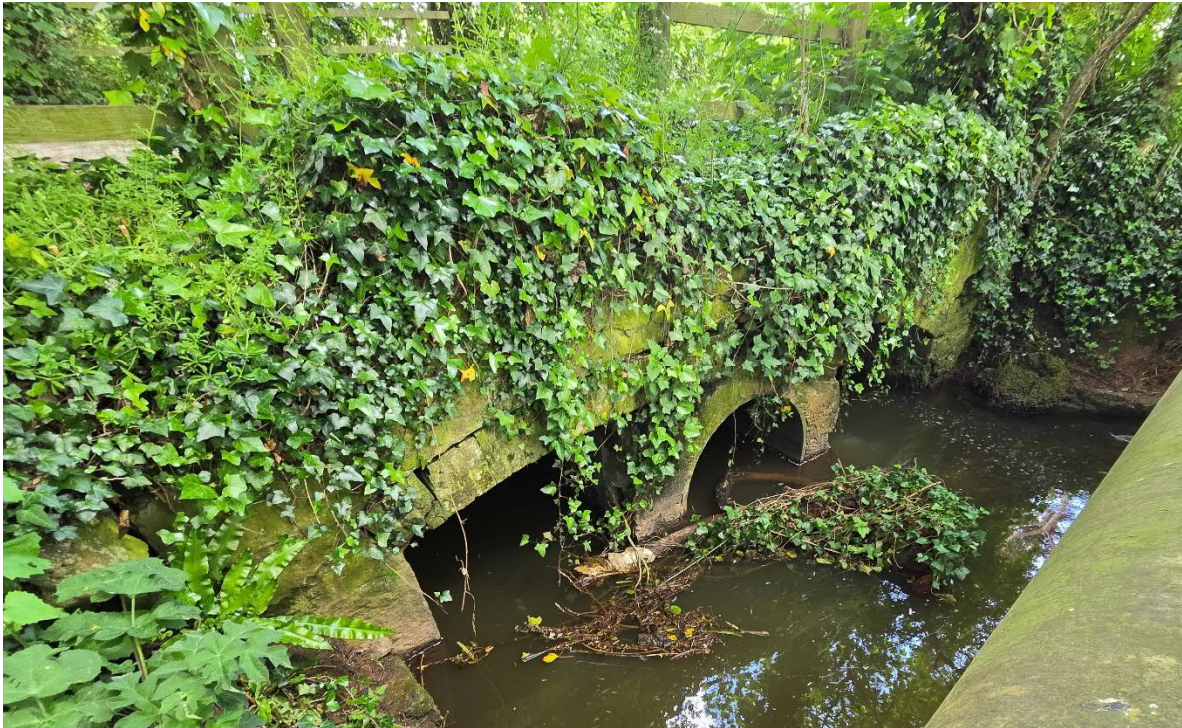
Figure 3: Bridge southern elevation.
