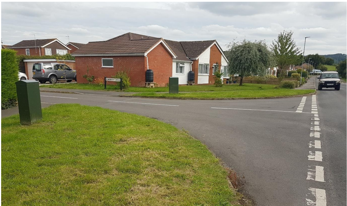
25 Verge at jnc of Swains Lane & Elworthy Drive - ///outfitter.fuse.legroom
