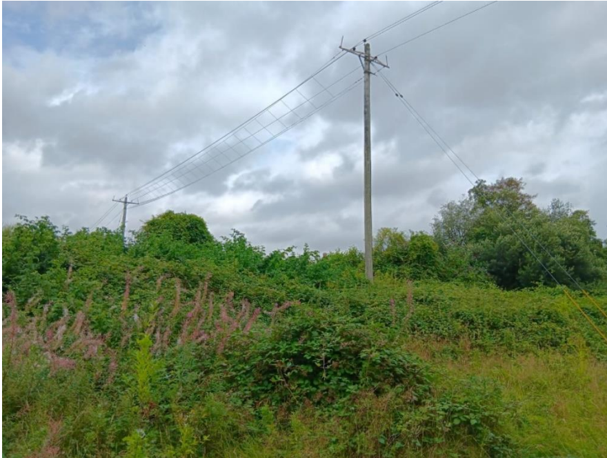
Photo 3: Northern planting area (cpt 1): power distribution lines across cpt 1.
